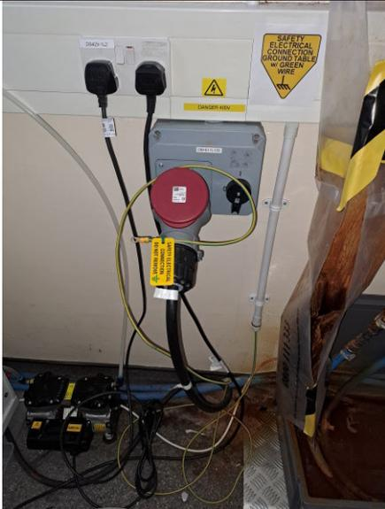
F11 grounding wire connection at wall
