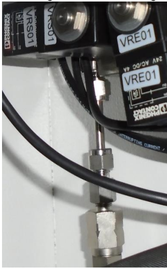
VRS01 valve and one-way valve.
