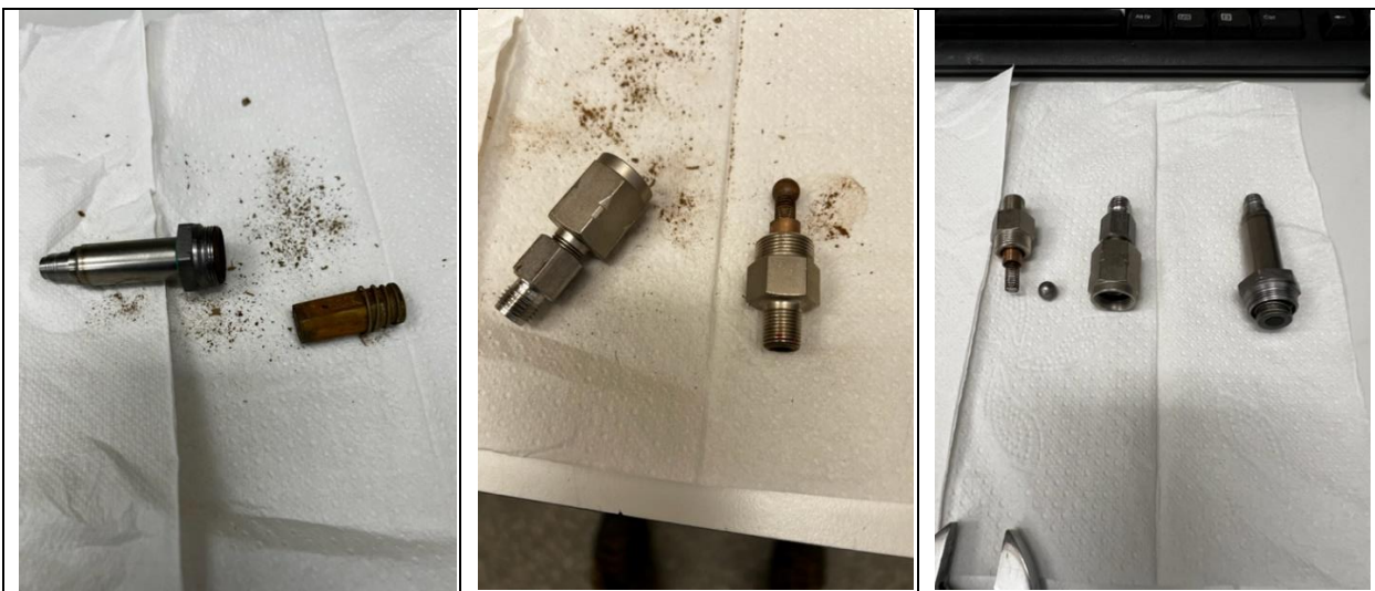
Before and after for VRS01 (left) one-way valve (centre), and cleaned parts (right).
